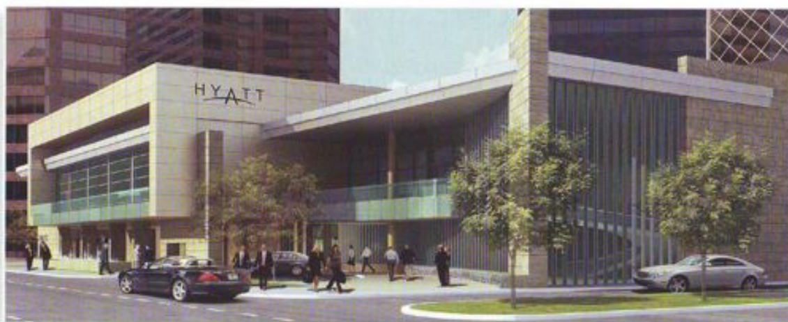
New owners are investing $275 million to return the 1,193-room Hyatt Regency New Orleans to the market next year.
